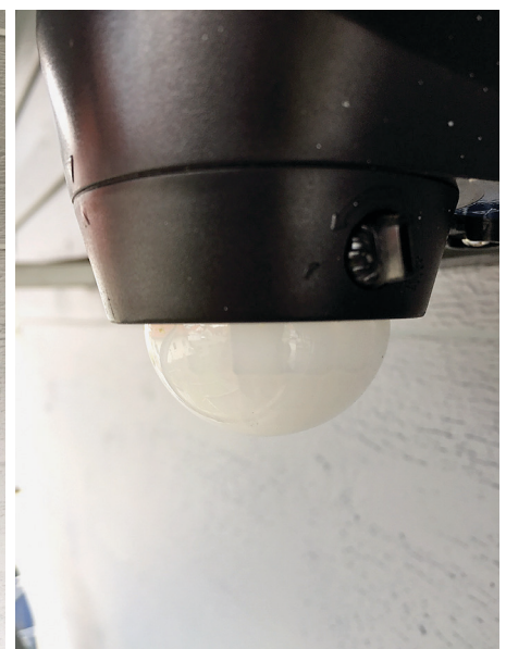
Figure 2. Automated light that is reactive to motion in the dark. Configuration allows the setting of thresholds for sensors and timings. Interventions prolong or terminate the light exceptionally.
